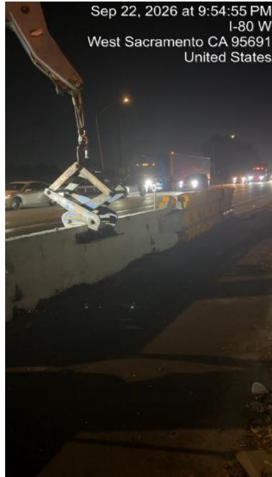
Removing K-Rail
