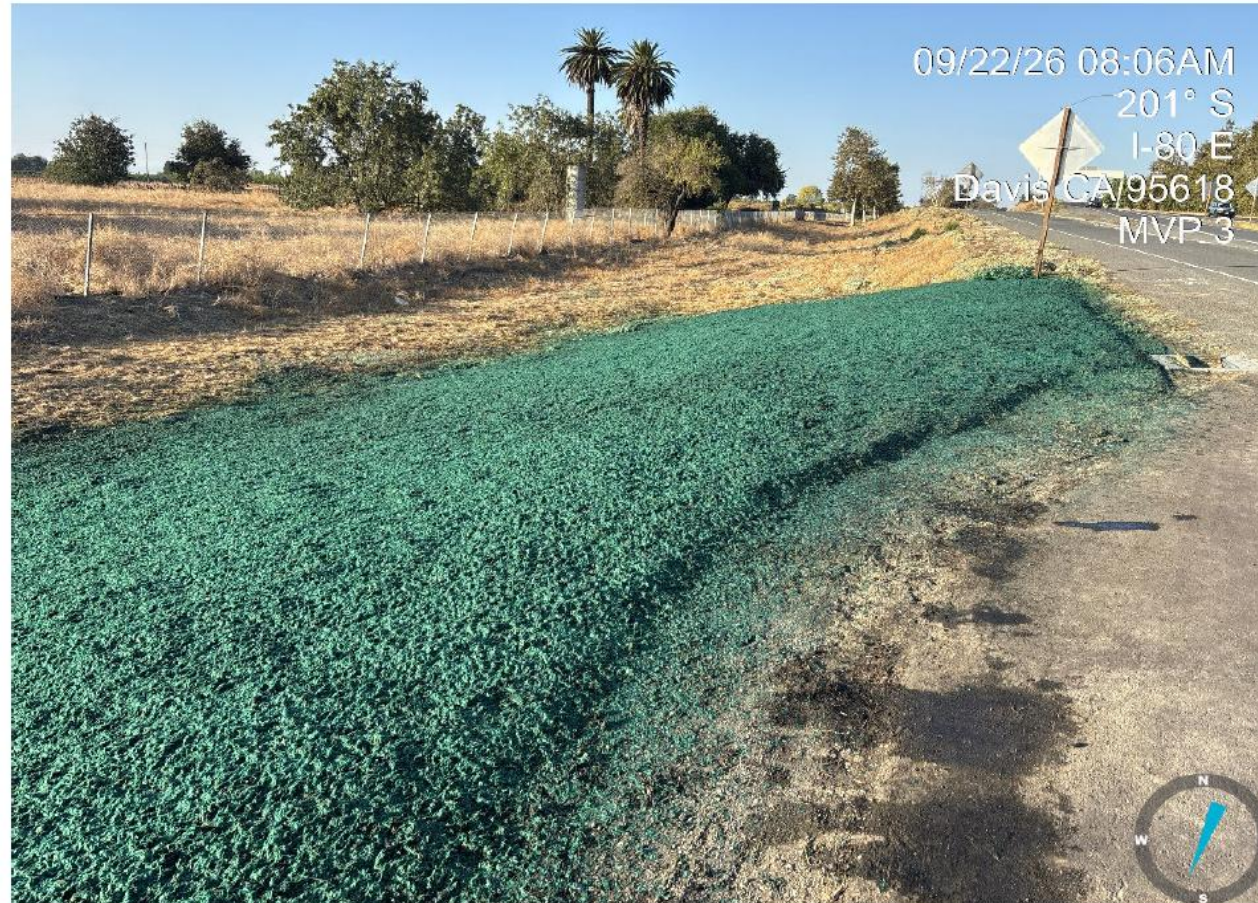
Installing Erosion Control
