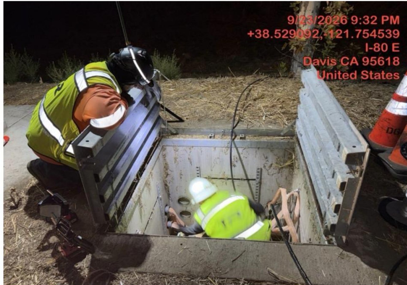
Installing Microwave Units
